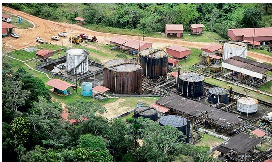
Figura 229: Andoas Station – Audit Point
