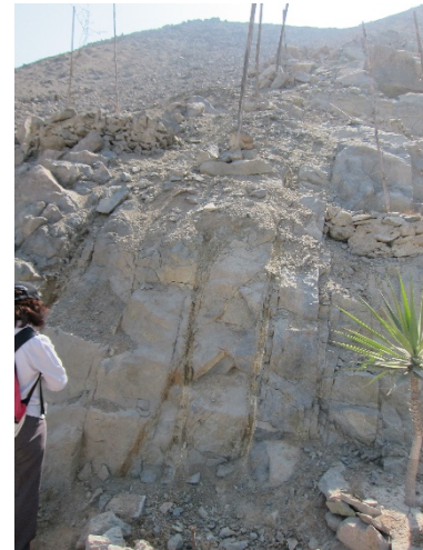
Figure 12. B2 portal: intrusive rocks, faults parallel to the excavation.
