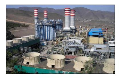
The Ventanilla Thermoelectric Plant was using natural gas from Camisea under the simple cycle system; That is to say, natural gas entered its two turbines, where a combustion originated whose force moved an axis acting on a generator that produced electric energy.
